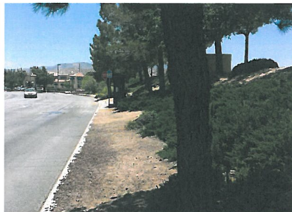
Area for new sidewalk
