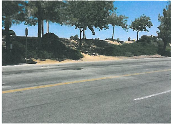
Area or AC street paving (one lane width) to be replaced per civil item 1
