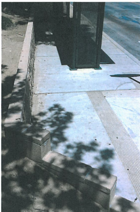
Existing retaining wall to be removed and replaced per civil item 1
