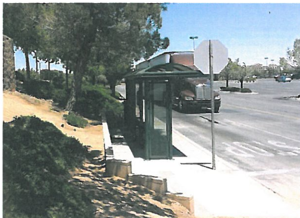
Existing retaining wall, shelter to be replaced
